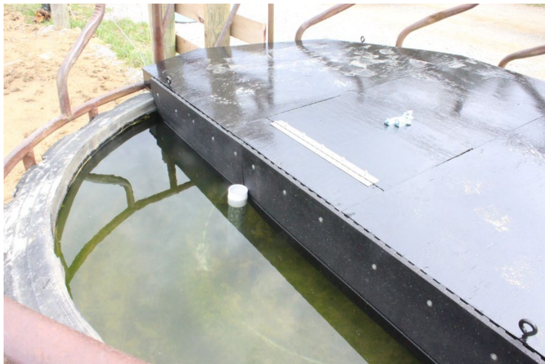
Figure 7. The top cover provided conveniences like a hinged door to monitor the float. Threaded eyes were installed to facilitate lifting and placement.
