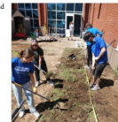
School Garden Construction at West Jessamine Middle School in Jessamine County
