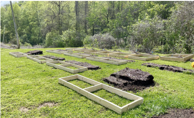
School Garden Bed Construction at W.B. Muncy Elementary in Leslie County
