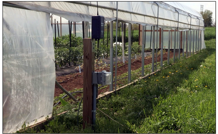
Screen shot from video by David Stalion, UK Ag Communications Sidewalls can be rolled up to provide ventilation.
