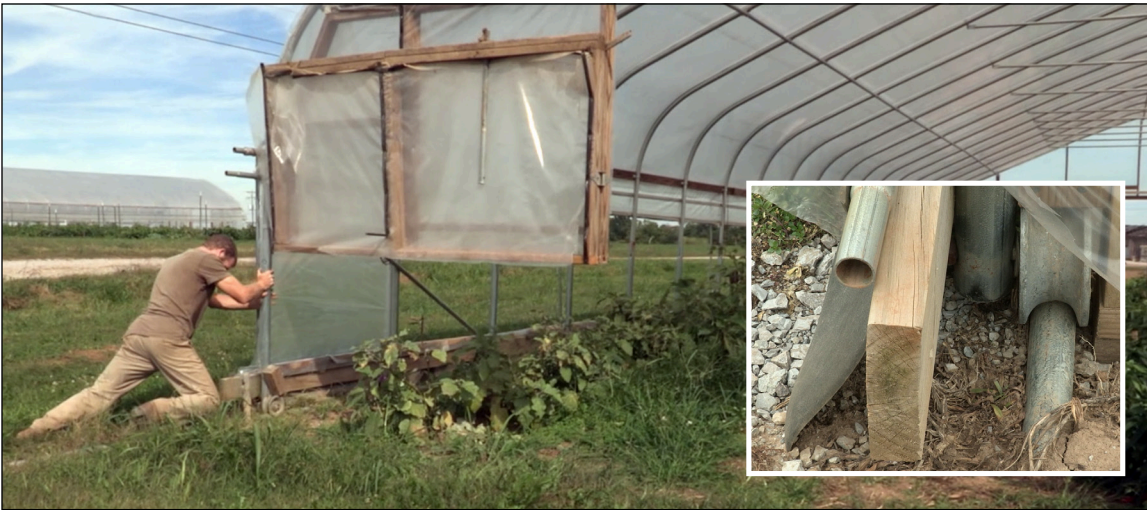
Moving a high tunnel using castors (inset) that roll along a galvanized round pipe below them.
