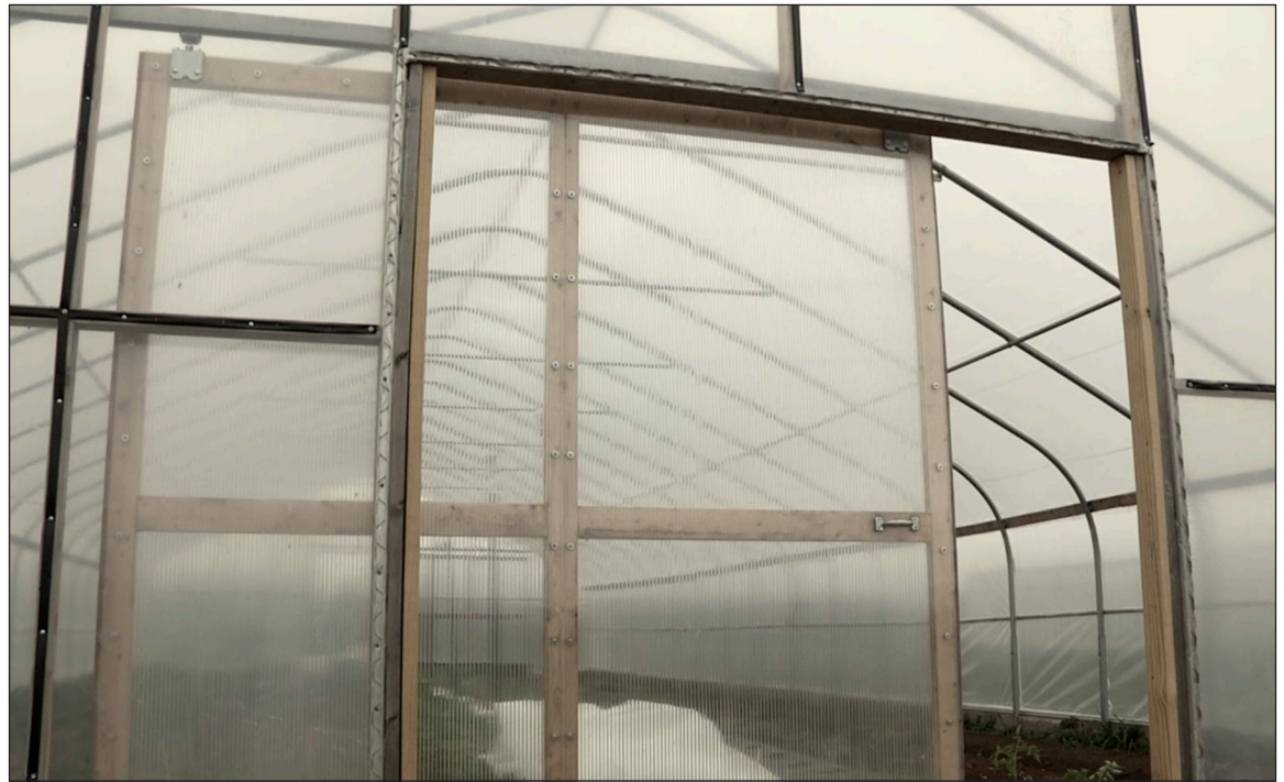
A sliding door on the endwall of a gothic high tunnel.
