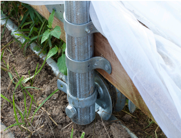
Above: two different kinds of rail system. First a “v” shaped track and second a round pipe rail. Both systems work with casters. Right: the tip of a ski system. This approach uses no rails and instead slides along the ground. Photos: Brett Wolff
